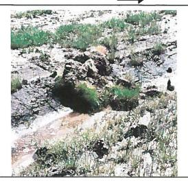
Someone deposited sod in the drainage ditch south of Lincoln St. This practice can lead to a blockage in the drainage which would affect everyone upstream with possible flooding. Please <u>do not</u> place anything in the drainage channels (including rocks), as the Town is prone to flooding and these drainage channels help to keep a clear flow through the community. (<u>picture above</u>)
